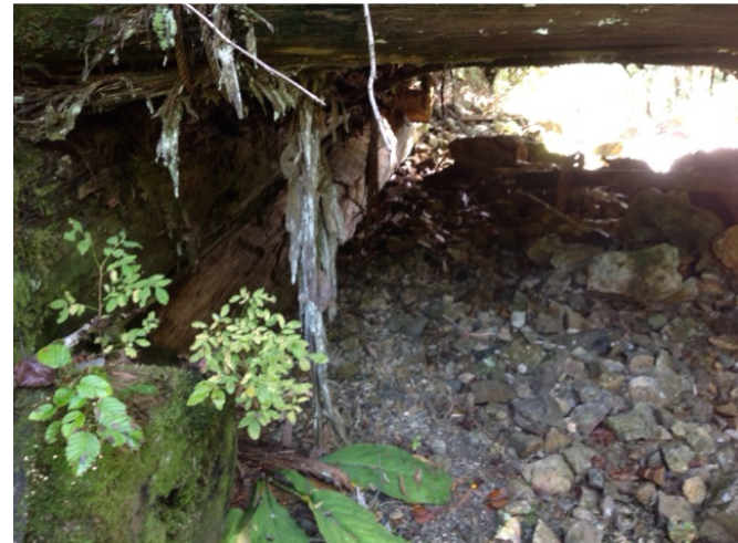
Left Bank Abutment when facing downstream
