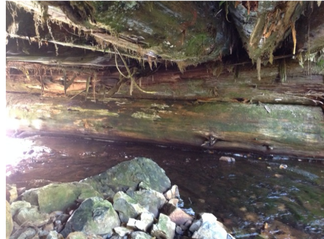
Right Bank Abutment when facing downstream
